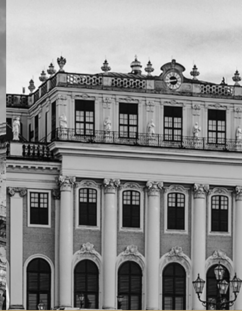
SCHONBRUNN PALACE Boroque architecture
